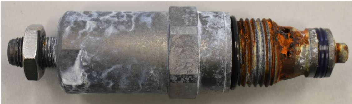
Sample after 1,008 h – white corrosion on the 25 % of evaluated surface
